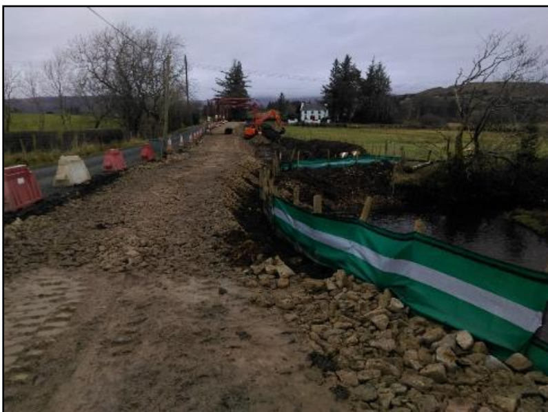
Plate 47 Looking west along ducting route
