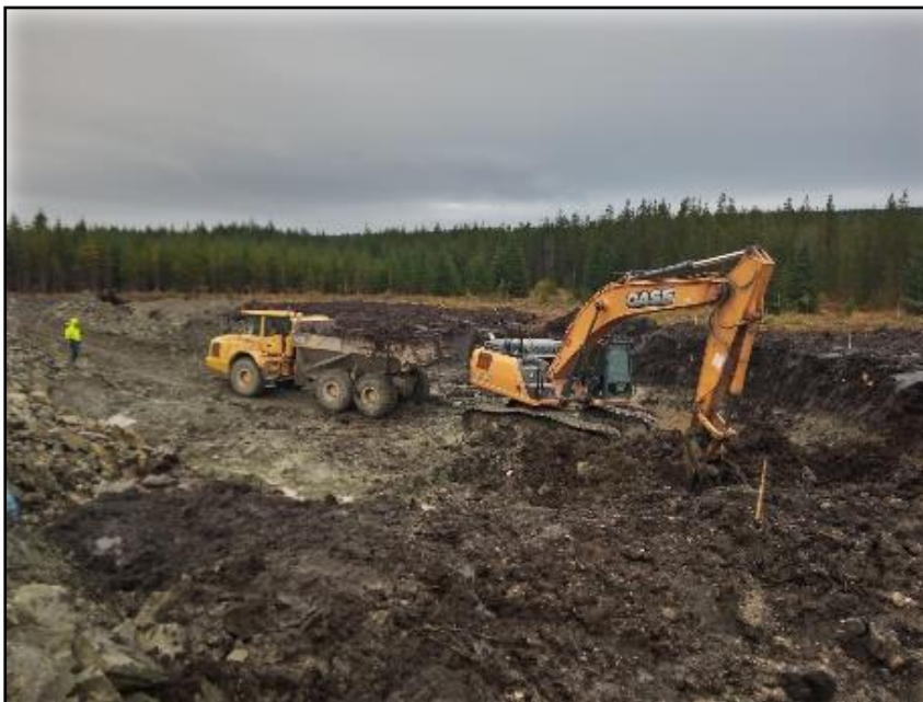
Plate 34 Looking east at T18 base excavation
