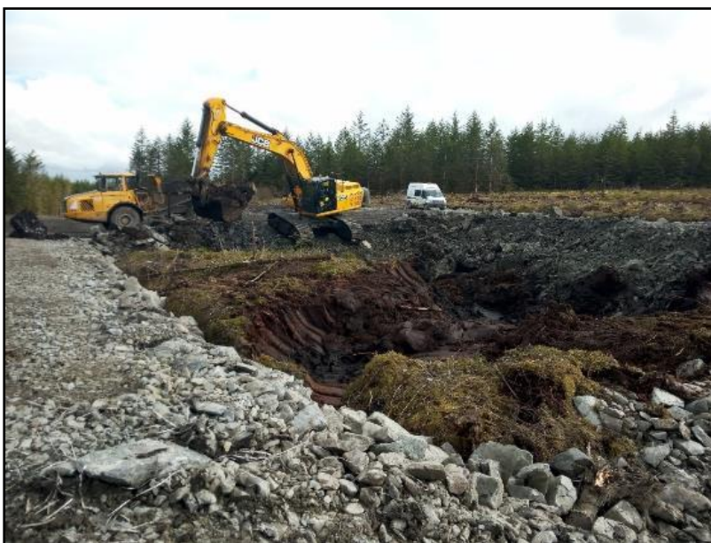
Plate 14 Looking northeast at T5 during peat excavation
