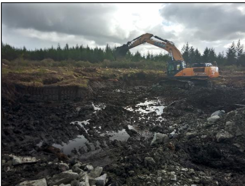
Plate 12 Looking east at T4 during peat excavation
