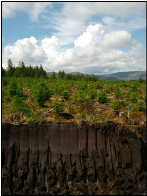
Plate 17 East-facing section of peat during excavation of road to T8
