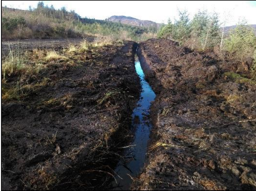
Plate 40 Drain north of substation
