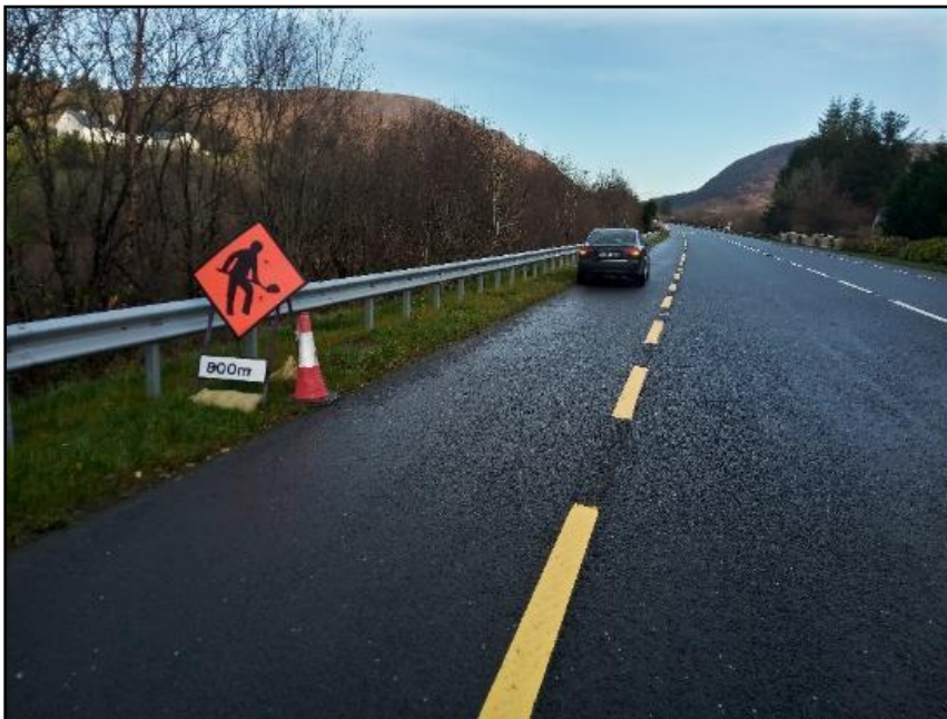
Plate 50 Looking north at site of DG094-026
