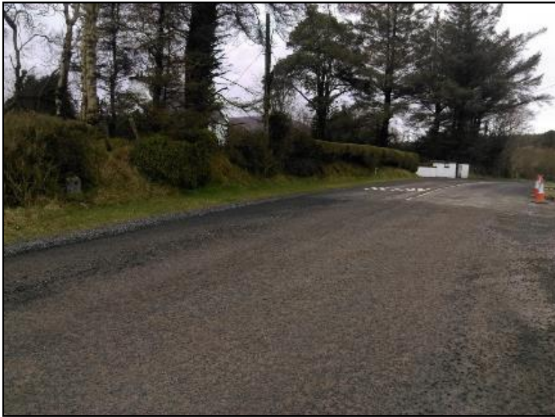
Plate 53 Looking northwest showing milestone (left) and nearest point of cable works (marked by cones at right)
