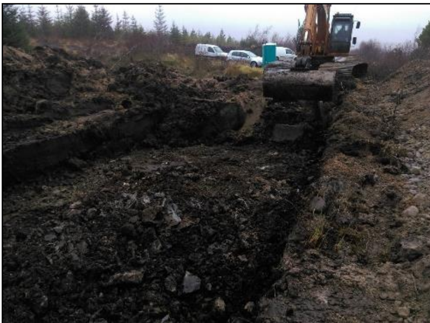
Plate 45 Peat excavations at compound site
