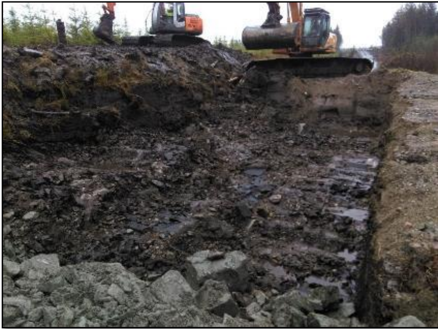
Plate 6 Road between first borrow pit and temporary compound
