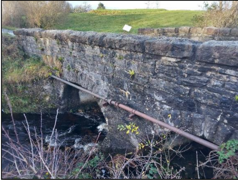
Plate 51 Looking west at road bridge NIAH Ref. 40909424
