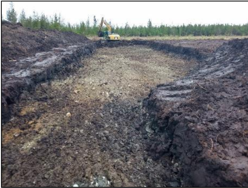
Plate 31 Looking east at excavation of T17 Hardstand
