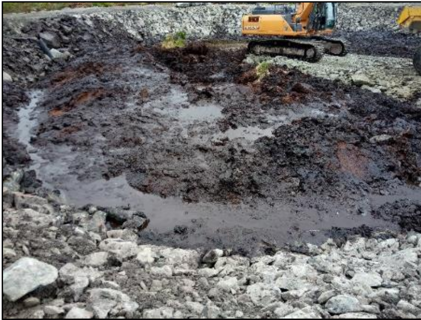
Plate 11 Looking south at turbine base during peat excavations at T3
