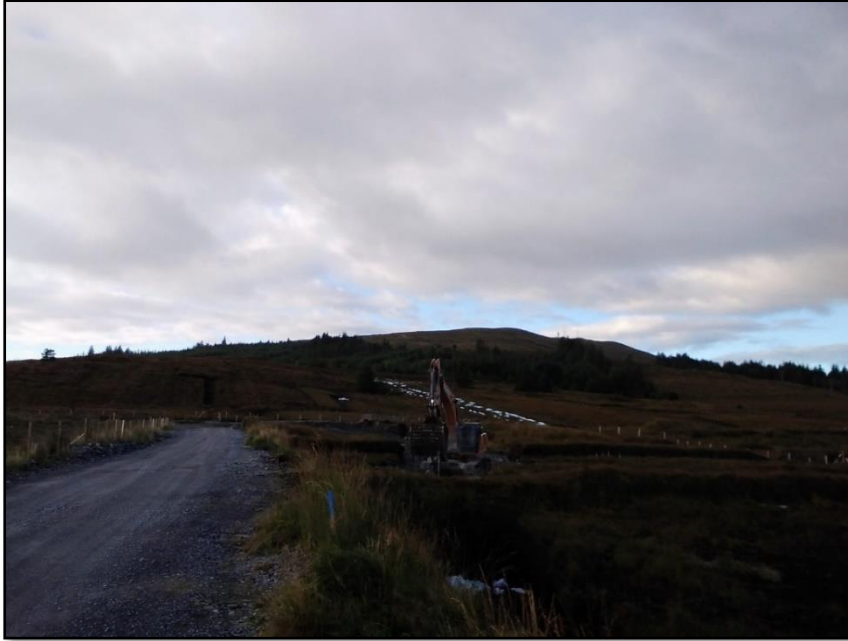
Plate 56 Looking east at Site Access Road Realignment
