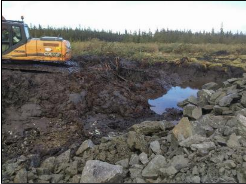
Plate 21 Looking north at peat excavations at T10
