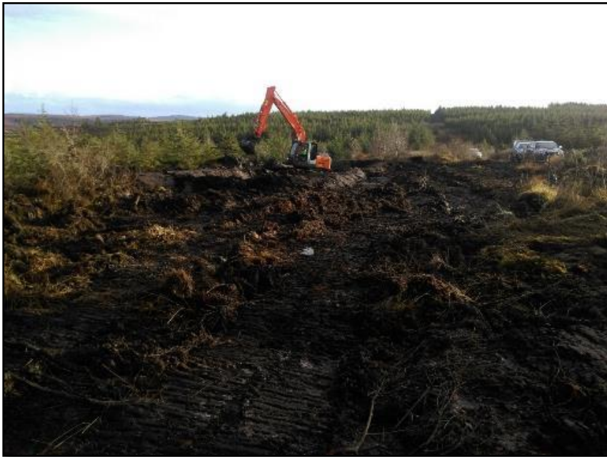
Plate 44 Peat excavations at site of substation
