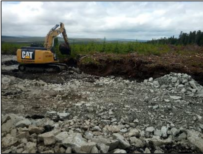
Plate 22 Looking north at hardstand excavation and fill at T11
